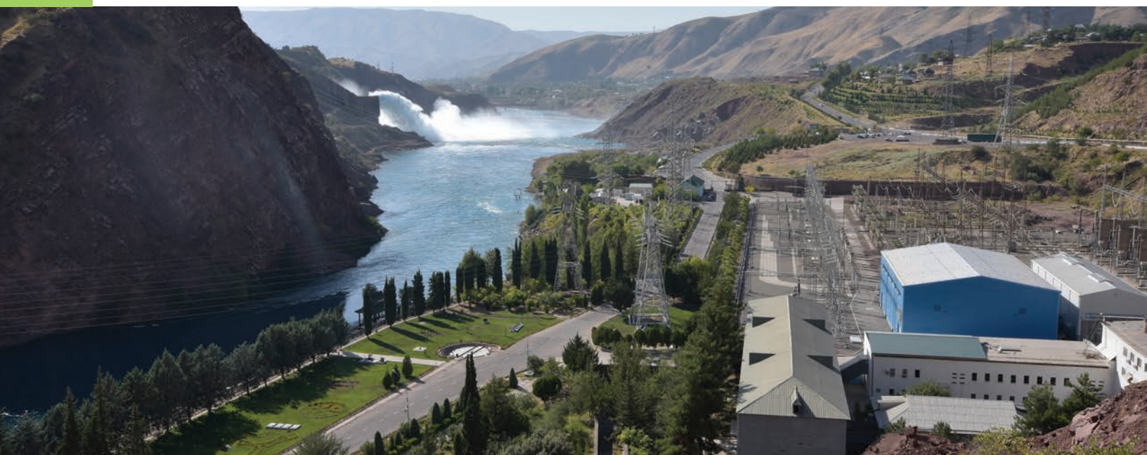
Nurek hydropower plant in Tajikistan. Photo: ADB.
